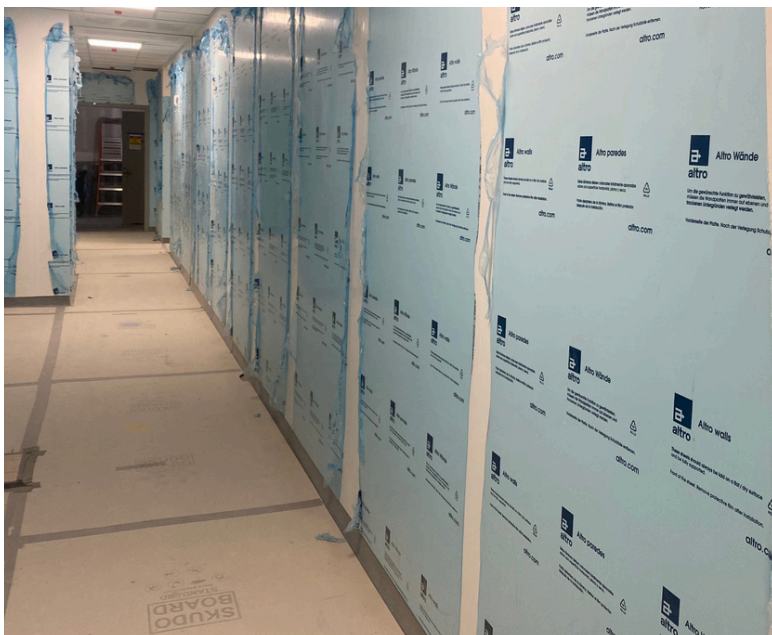
SRI installation of Altro hygienic wall coverings for hospital pharmacy
